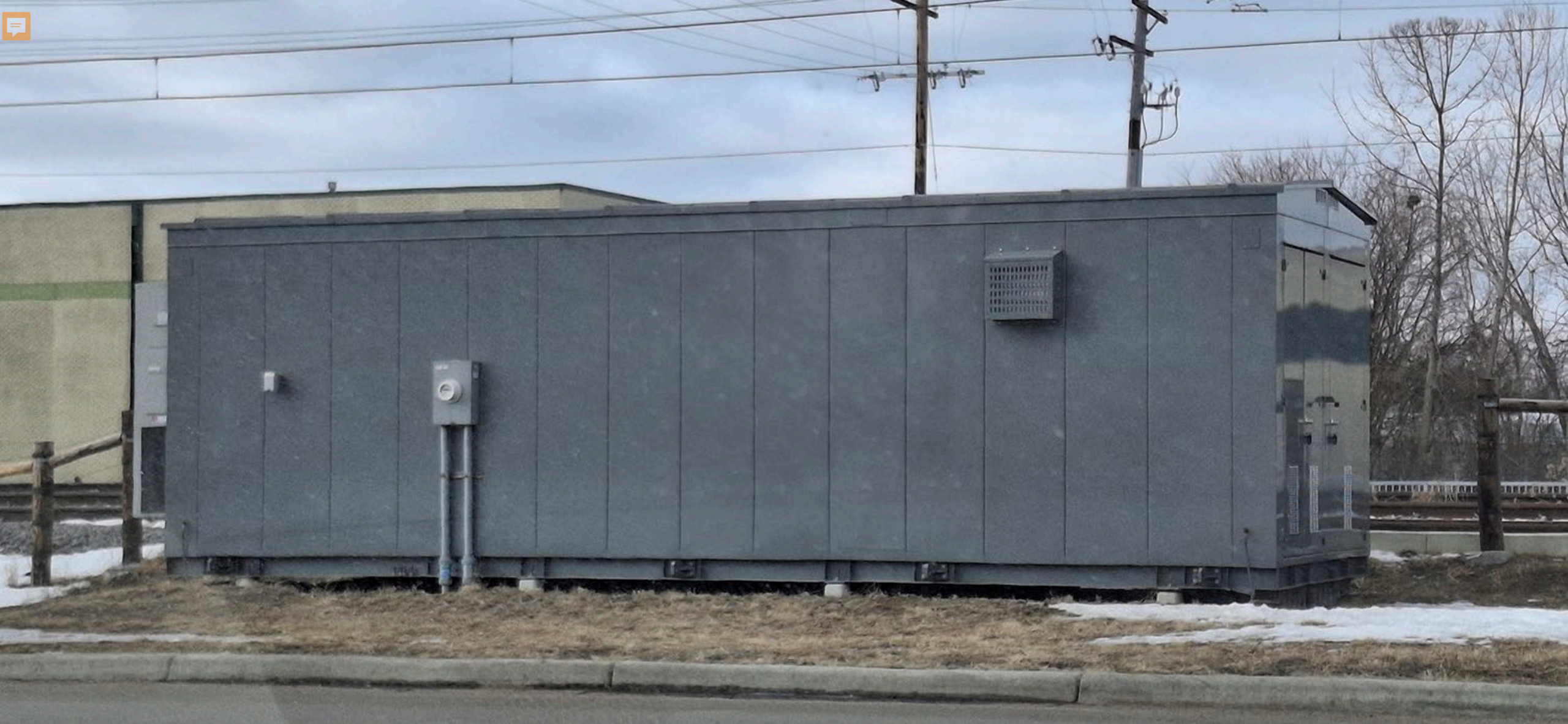
2026 New Artwork Green Line Extension Signal Houses
