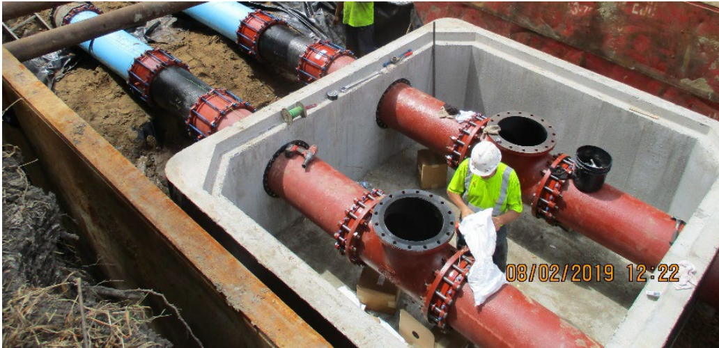
Contractor installation of 7071 Forcemain
