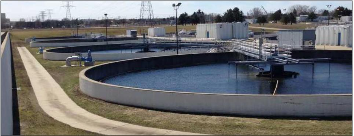
Blue Lake Water Resource Recovery Facility (WRRF)
