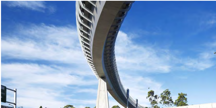
Figure 10: Steel box girder pedestrian bridge. (Photo from KI Studios).
