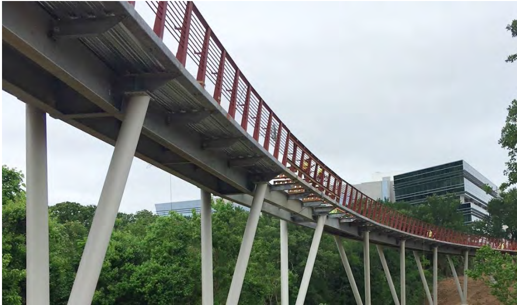
Figure 9: Steel plate girder pedestrian bridge. (Photo from Southern Steel Engineers).
