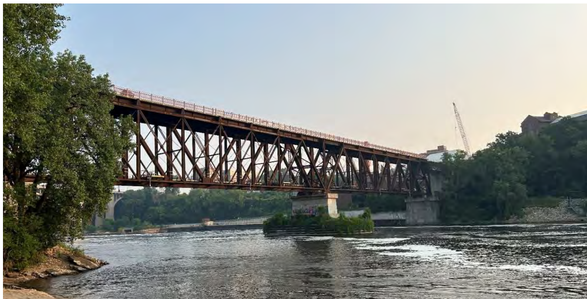
Figure 8: Bridge 9 steel deck truss over the Mississippi
