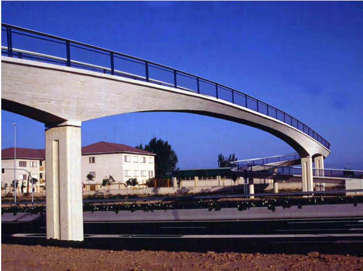
Figure 13: Pedestrian bridge in Alicante, Spain, showing variable-depth concrete box girders
