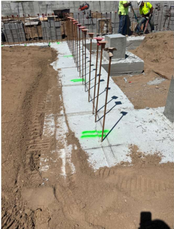
July: Gunnar working on underground electrical and installing electrical in the masonry walls.
