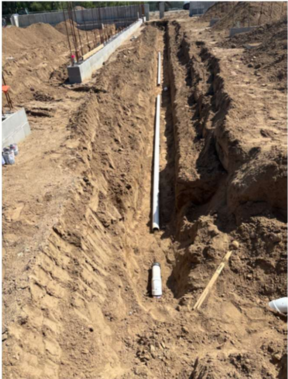
July: Gunnar working on underground electrical and installing electrical in the masonry walls.
