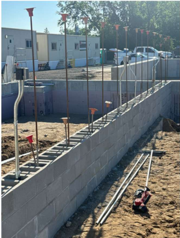
July: Gunnar working on underground electrical and installing electrical in the masonry walls.
