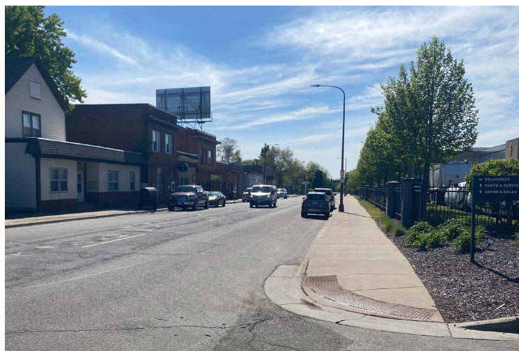
View: Unsignalized intersection of E 7th St and Duluth St, looking west towards mixed use land uses.
