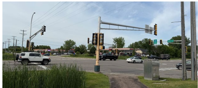
INTERSECTION WITH COUNTY ROAD 92 (MAIN STREET)
