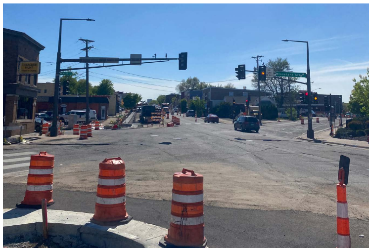
View: E 7th St, N Mendota St, and Minnehaha Ave E, signalized intersection looking southwest during construction.
