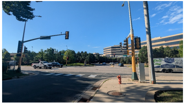
Photo: Newton Avenue at 76 th Street, facing South, June 23, 2026
