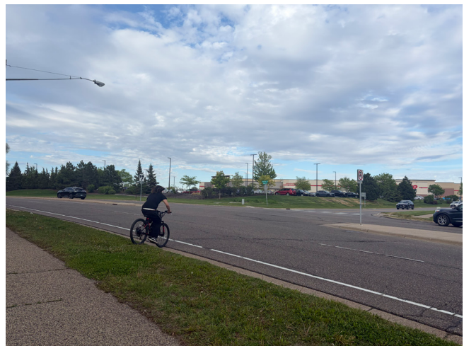
Curb ramps and a median island will be constructed at 141st Street to provide for safer pedestrian and cyclist crossings
