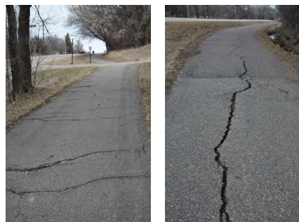
Trail to be reconstructed 10' wide with 2-3' clearzones
