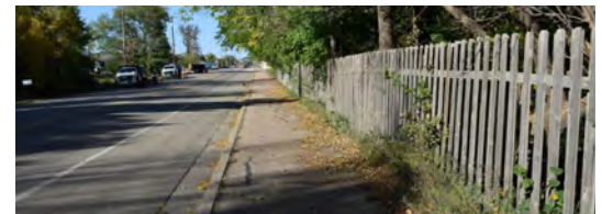
Trail to be reconstructed 10' wide with 2-3' clearzones
