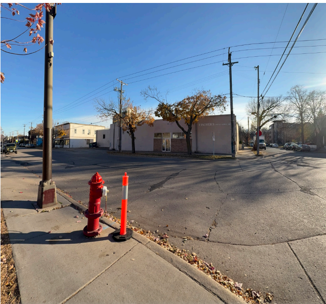
Existing conditions include deteriorated pavement, uneven or heaved sidewalks, and multiple obstructions within the public right-of-way; all of which create safety hazards for pedestrians
