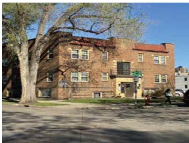
Existing conditions: Intersection of 18th St
