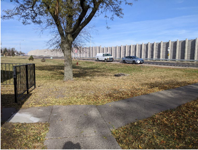
Figure 1 A portion of the one-third mile sidewalk gap along L'Orient
