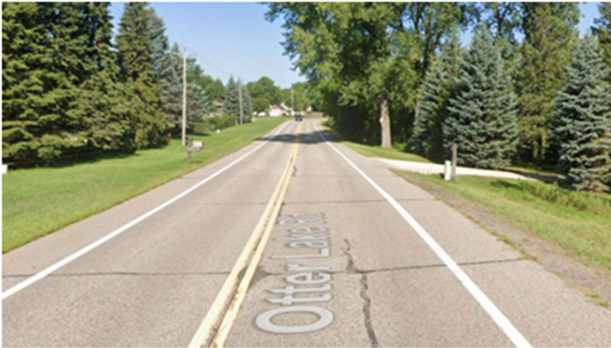
Image 2: Existing Road – Taken at 5630 Otter Lake Rd (facing North)
