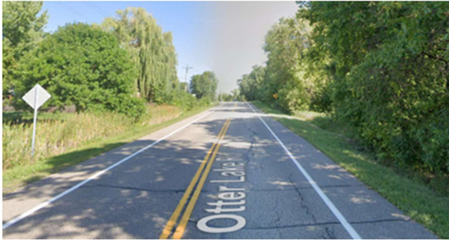
Image 4: Existing Road – Taken at 5690 Windmill Dr (facing North)
