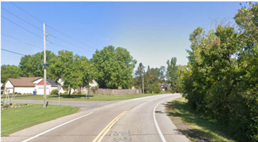
Image 3: Existing Road – Taken at Brandwood/Otter Lake Intersection (facing North)
