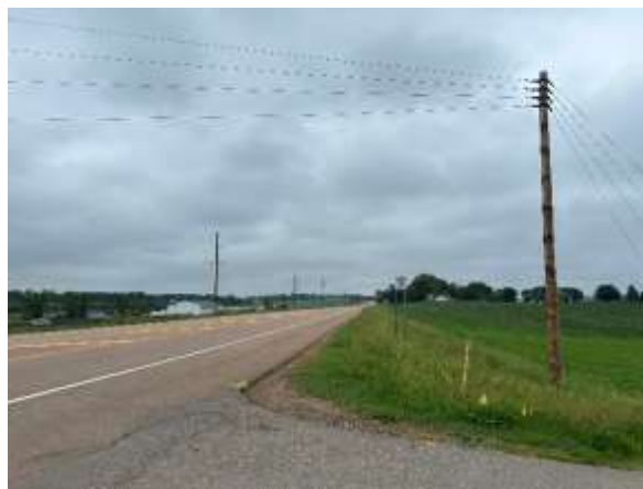
(Figure 1: Looking North along Highway 10 (Waconia Parkway))
