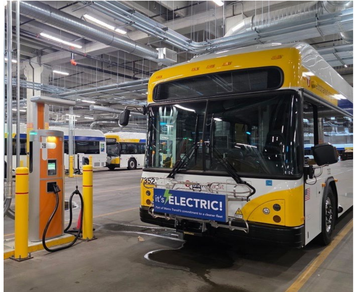
Gillig electric bus parked next to a ChargePoint plug-in dispenser at North Loop Garage
