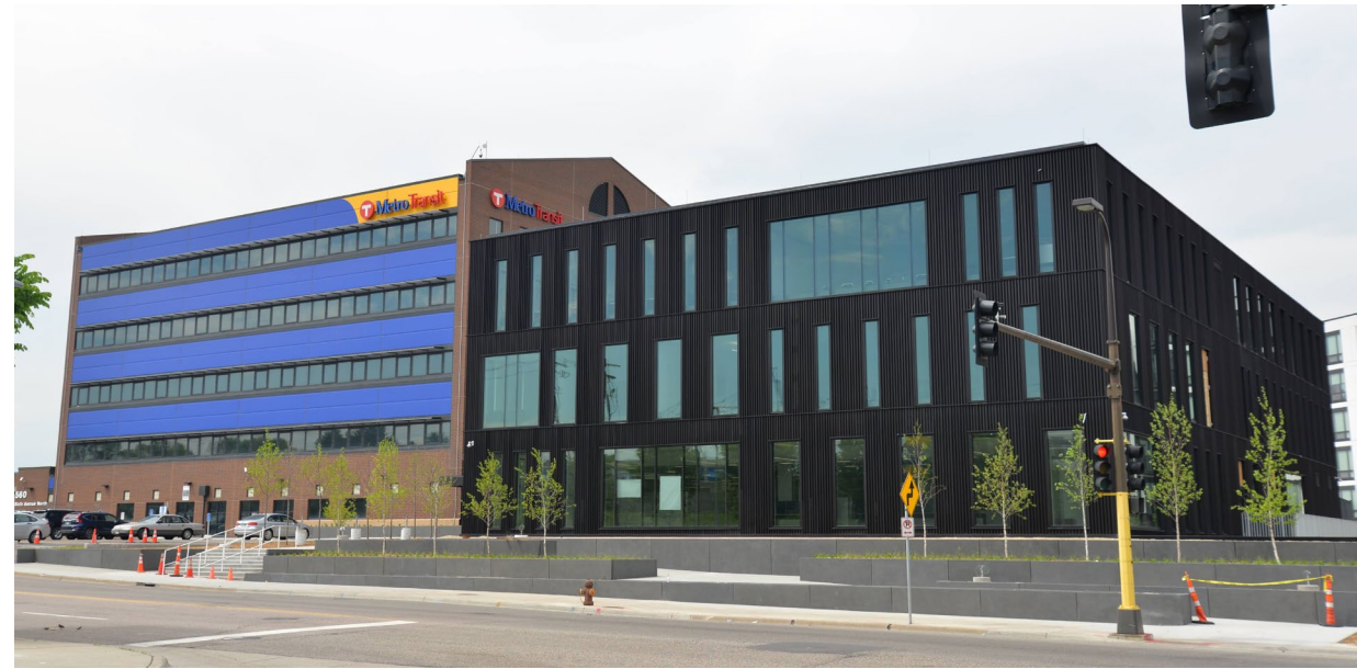
Fred T. Heywood Office Building and Garage (Image source: Metro Transit)
