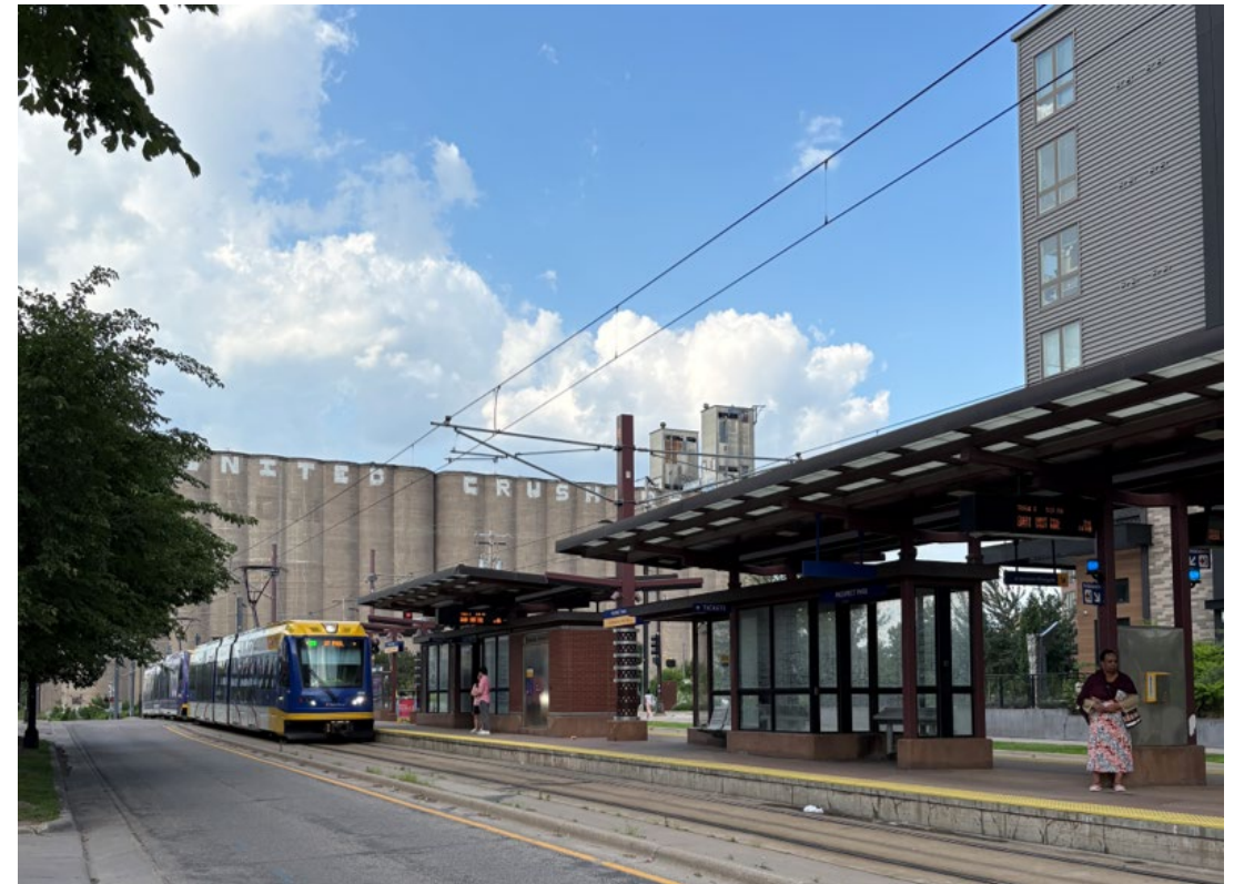
Green Line, Prospect Park Station (Image source: SRF Consulting)
