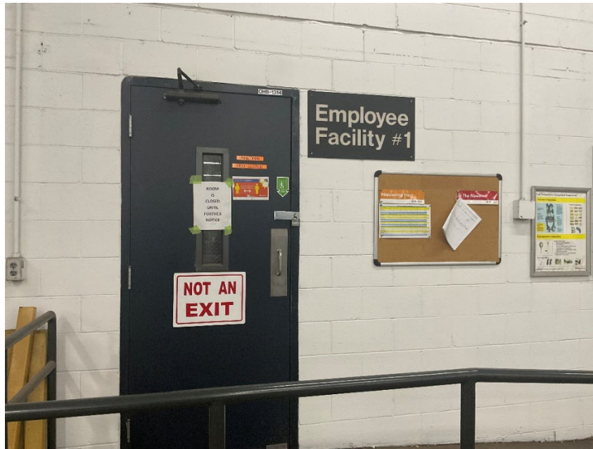
Image A: Interior view of the previously operational Overhaul Base lactation room.
